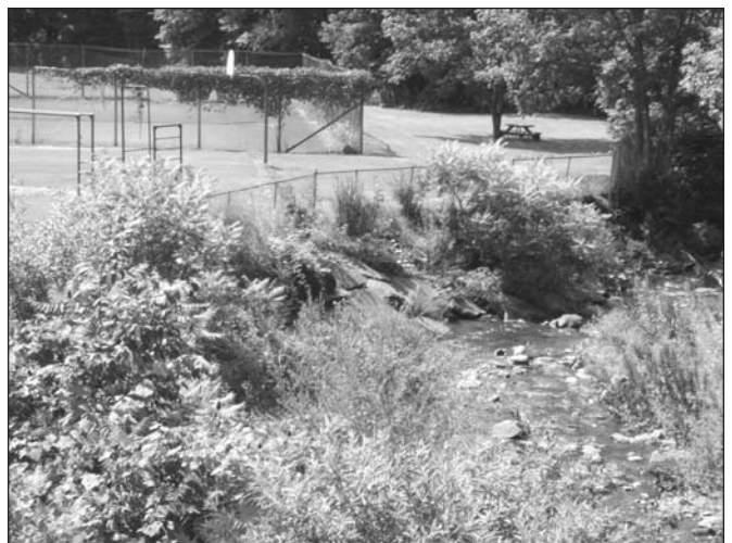
Birch Creek's bank is slip-sliding away in the vicinity of the Pine Hill community playground. A grant to the Town of Shandaken from the CWC's Stream Corridor Protection Program will armor and reseed the bank to prevent further encroachment on the park.
